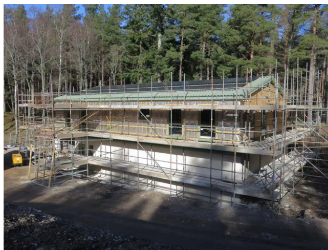
Aboyne and District Men's Shed nearing completion
