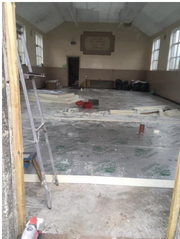
Fittie Gospel Hall - work in progress to install the new heating system
