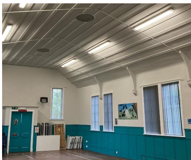
Figure 1. Leswalt Hall: photo shows new windows, door, blinds, LED lights, and paint work.
