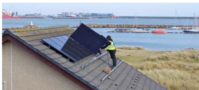
Solar panels being installed on the Clubhouse at Peterhead
