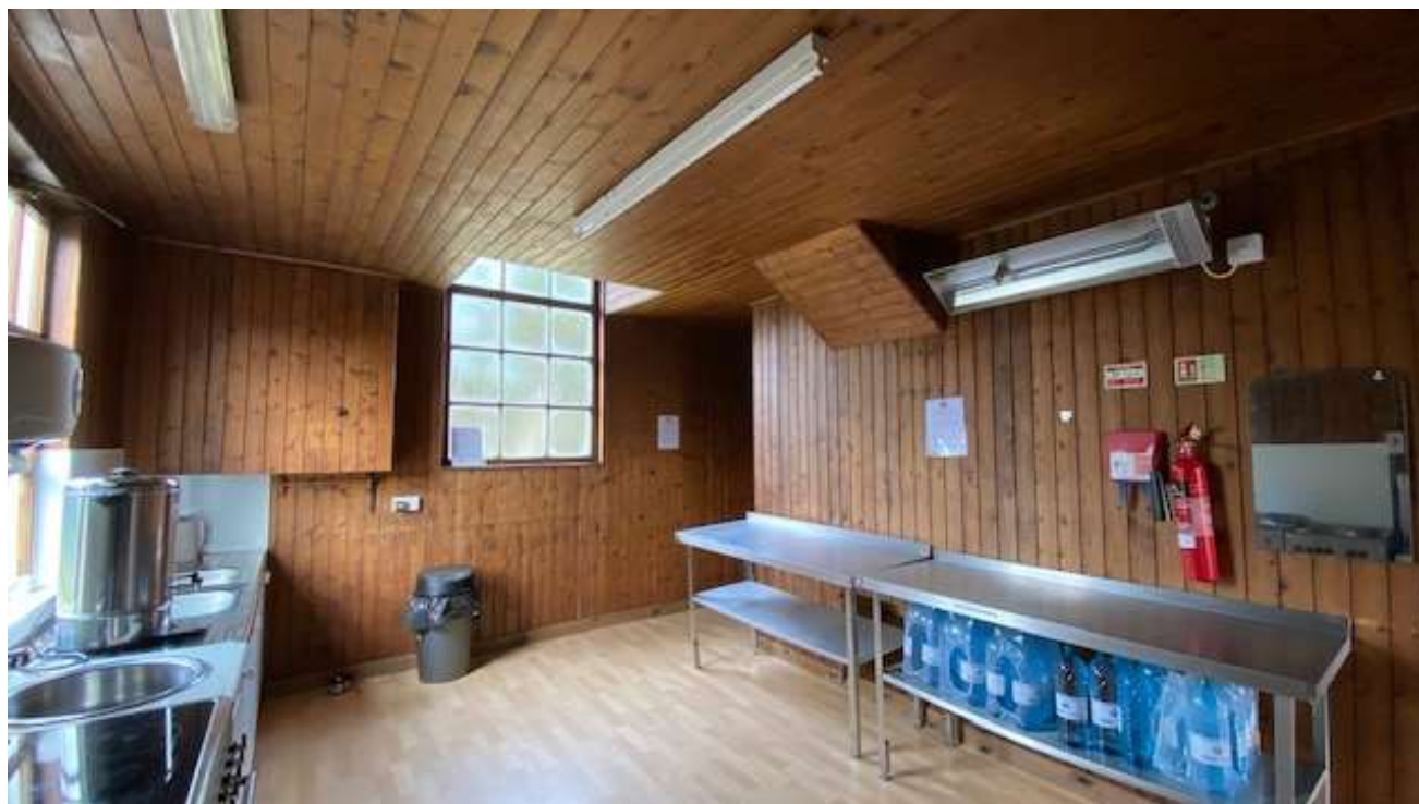
Photo: Kitchen before refurbishment
