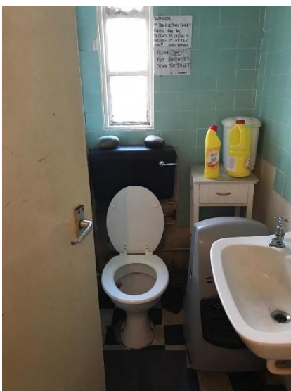
The current toilet facilities – 25/01/24
