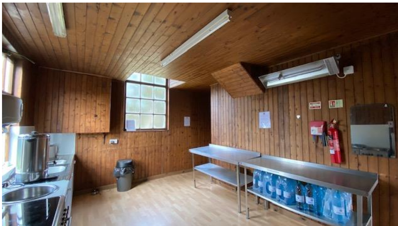
Photo: Kitchen before refurbishment
